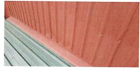
Also, the fasteners were installed incorrectly as they were to be mounted in the 'valleys' and not on the ridges as shown.
