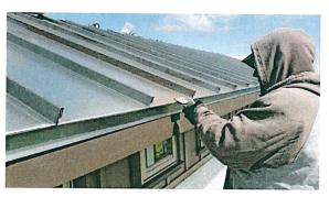
flashing with a clear path back into the roof...Here you can see where water ponds at the edge due to low pitch (see discolored spots.) Notice they put screws in or near the ponds.
